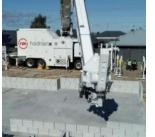
This robot, mainly mounted on trucks, and adaptable for tracks, barges, cranes, and other heavy vehicles, can lay brick over a large area with precision. This is possible thanks to its Dynamic Stabilisation Technology (DST), which allows Hadrian X to adapt to wind, vibration, and other external variables.
